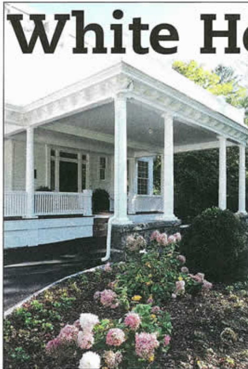
Peter Georgoutsas rebuilt the porte-cochere, reinforcing it with steel beams. Homeowner Katie Kahn says they discovered carpenter ants had eaten away at the original ceiling and was in serious danger of collapsing if it wasn't replaced soon.
