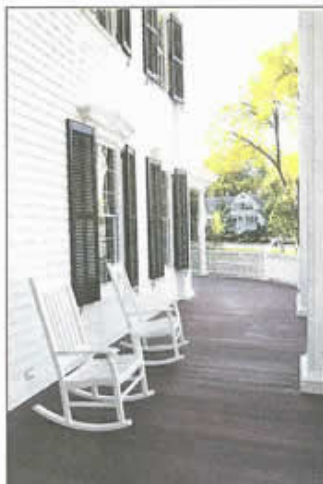
The large porch was completely rebuilt by Van-Go Contracting in Bergenfield. Owner Peter Georgoutsas custom-milled pediments over the windows and recreated the porch with mahogany wood.
